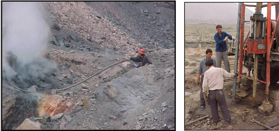
Figure 16 a and b Fire fighting by water supply (a) and drilling to inject synthetic foam (b)
