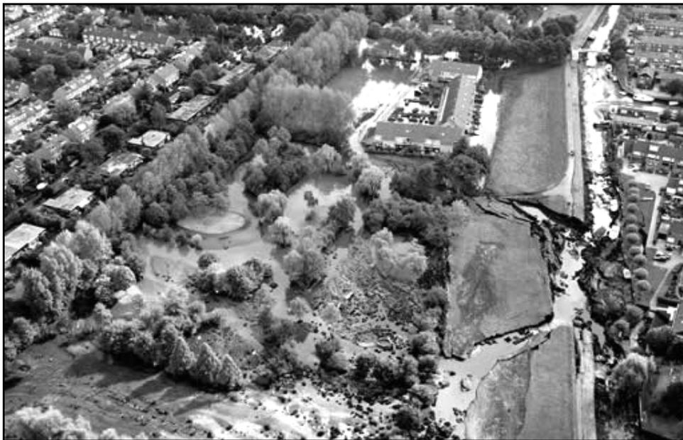
Like many other small dikes in the Netherlands, the complete dike consists of peat. Since peat has a relatively low specific weight, a peat dike has a higher risk of being pushed aside by water pressure than sand or clay dikes. This horizontal sliding is a rare type of failure mechanism. However, checking the stability of this dike using a simple computation makes clear how realistic the failure of a dike after a long dry period is.
