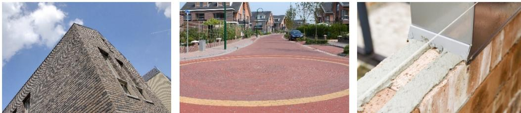
**Figure 20. From left to right: facing bricks, paving bricks, and inner wall bricks. Facing and paving bricks source: (KNB, 2020), inner wall bricks source: (Architectenweb, 2020).**
