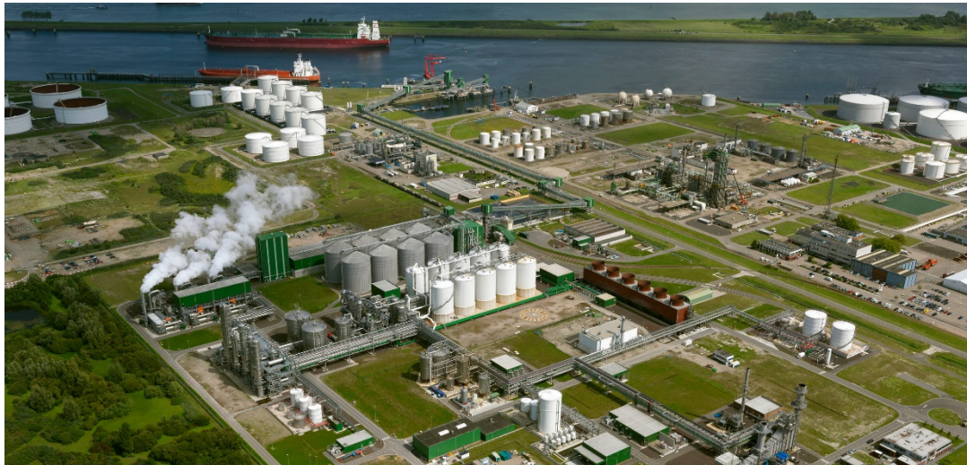
Figure 5. Alco Energy Rotterdam B.V. (Water talent, 2017)
