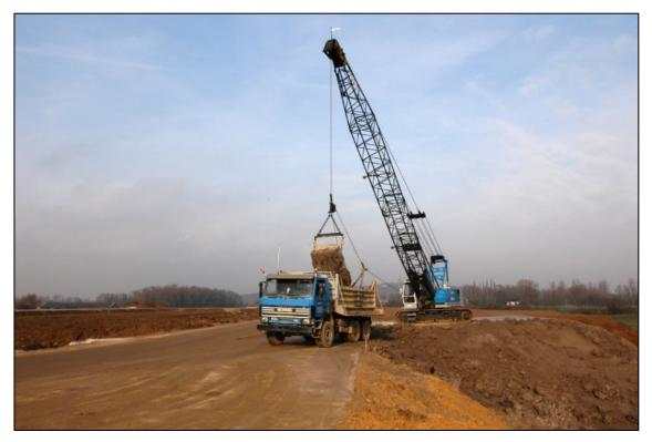
Figure 6. Storage yard (in Dutch 'kleidepot') where extracted clay is stored, often closely located to the ceramic plant (KNB, 2020).
