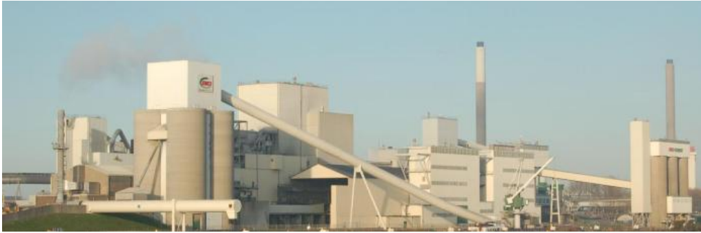
Figure 2 - ENCI IJmuiden industrial site
